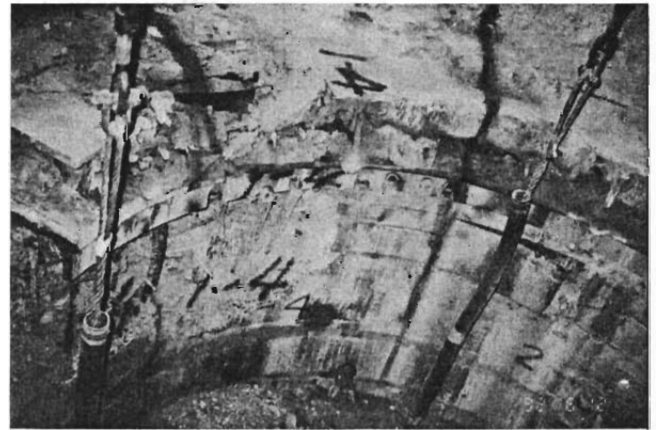
Photo 3 Demolition in Under Charging
